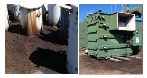
Figure 2.15 Soil contamination associated Figure 2.16 Damaged 69KV with discarded distribution transformers - Sophia Sophia
